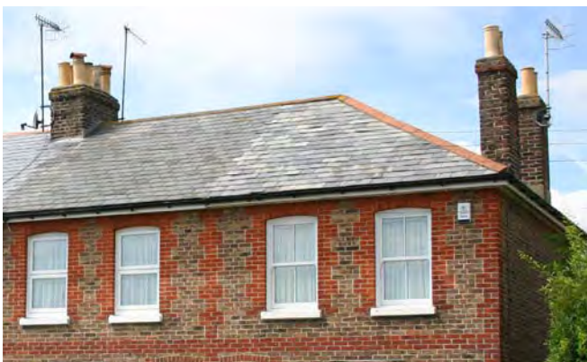
Hipped roofs and chimneys should be used to add variety to the roofscape.
