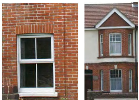
Arched brick headers and flat stone or brick headers are common in the area. Bay windows could be used on key buildings.
